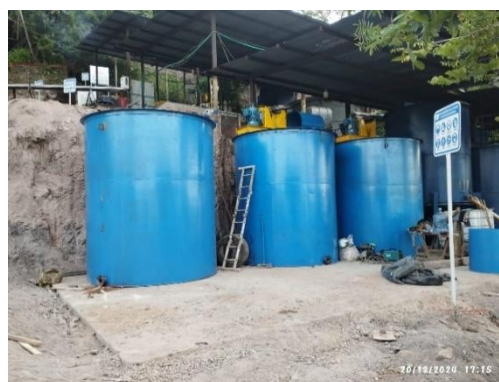
PHOTO 2 : NEW AGITATOR TANKS – SANTA BARBARA PROCESSING PLANT
