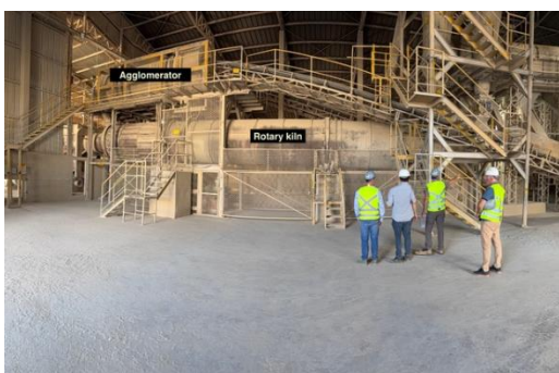
PHOTO 8 : ROTARY KILN DRYER
