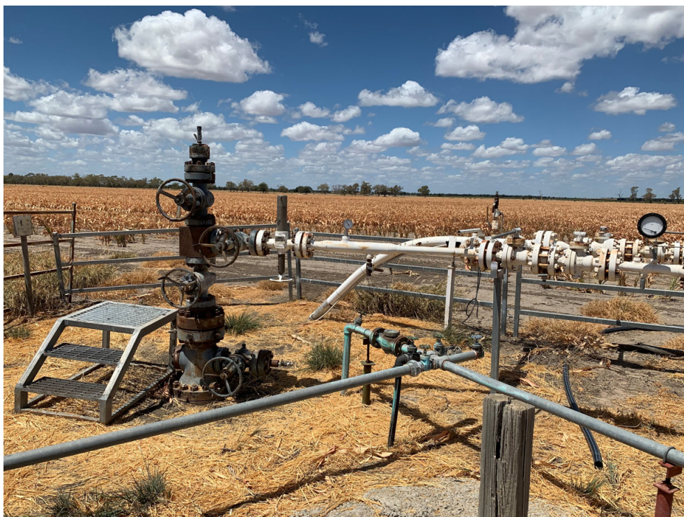
Figure 10 - Myall Creek #02 well head facilities
