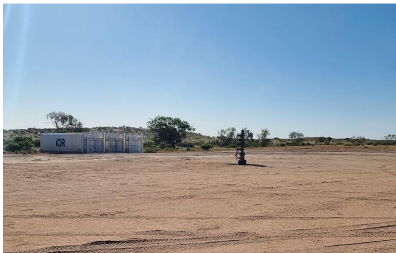
Figure 1: Kiwi 1 Wellsite post EPT
