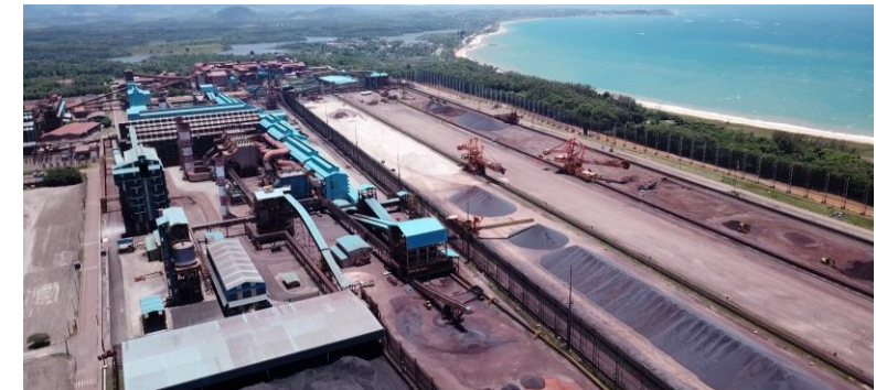
Ubu Complex: filtration and pellet plants, and port
