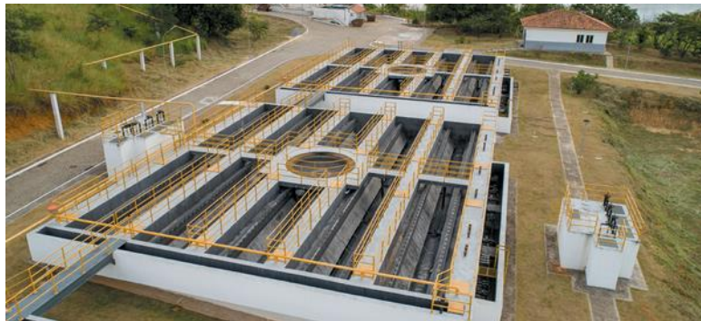
Sewage treatment plant, Colatina
