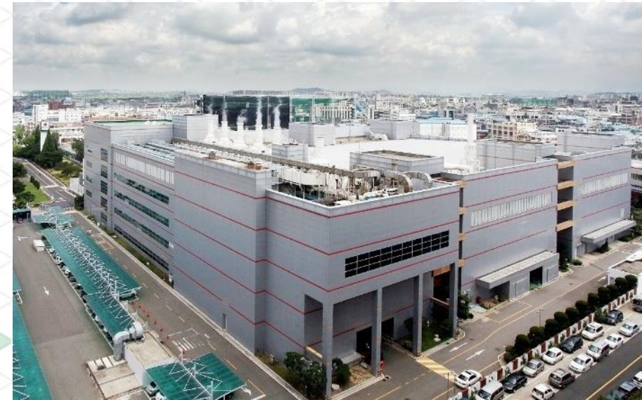
Above: a DB HiTek plant
