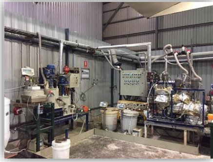
Phosphate Extraction Pilot Plant
