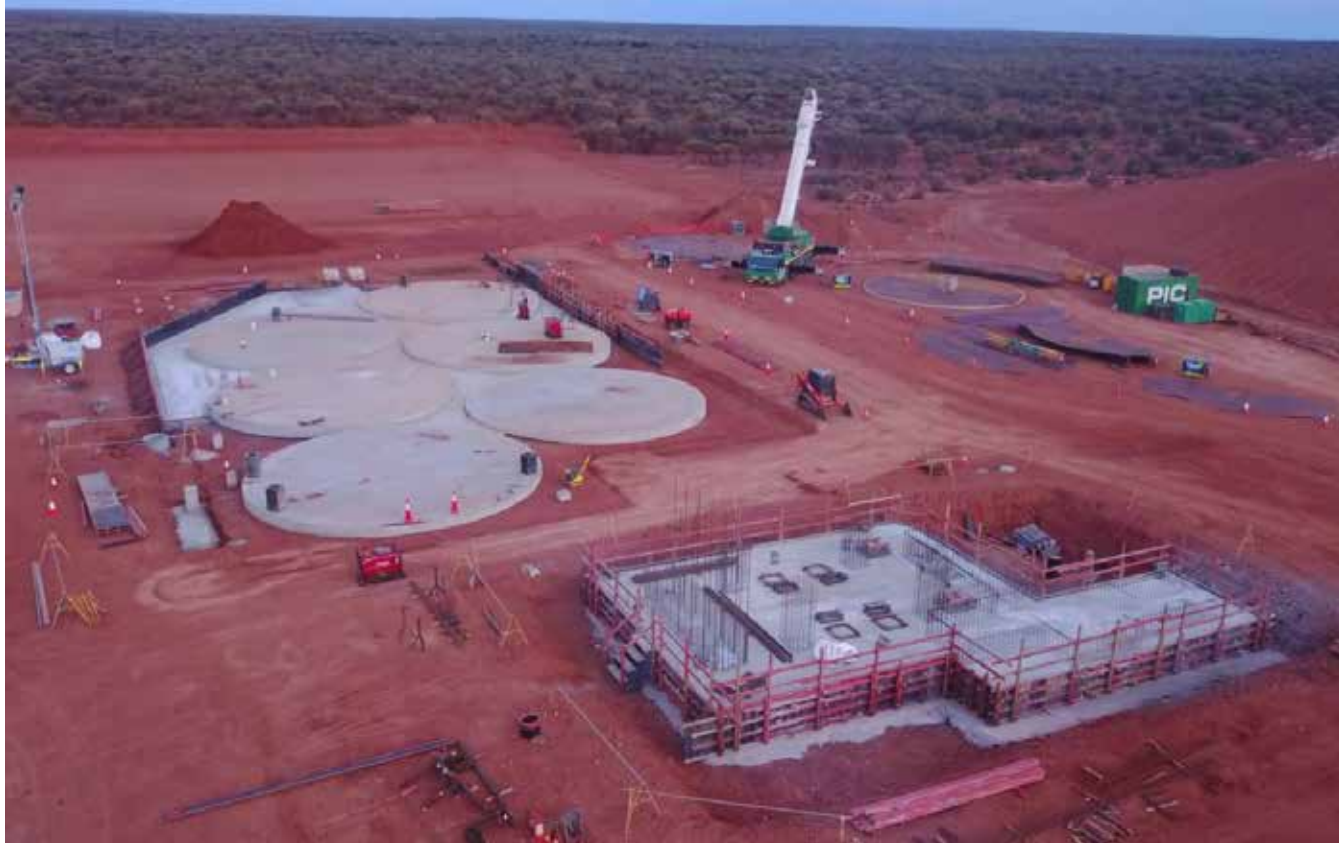
SAG Mill and CIL Tank Foundations
